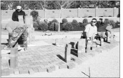
Pavers were laid by hand over an 18" gravel
