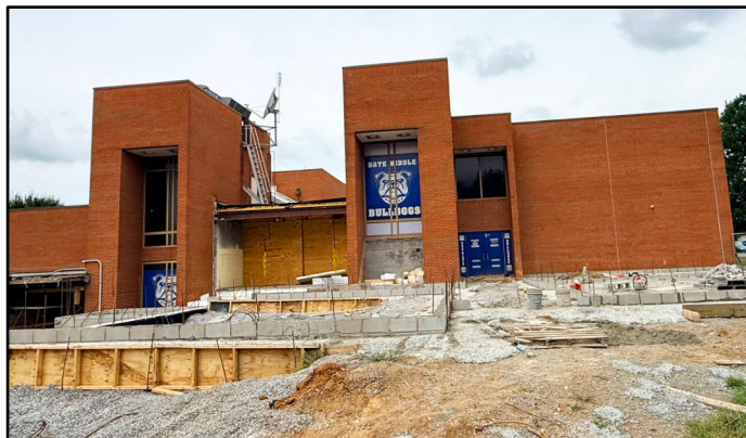
The Bookmobile will boost services during Bate construction.
